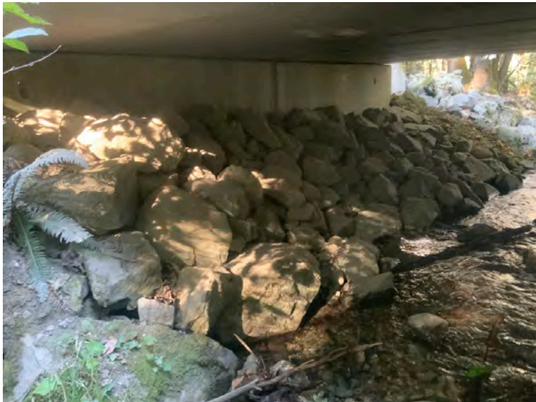
Left Bank Abutment when facing downstream
