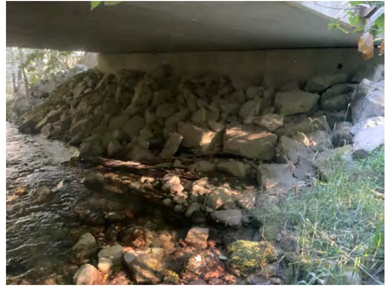
Right Bank Abutment when facing downstream
